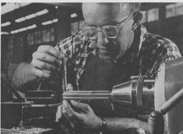
CHECKING LATHE WORK, Paul Chavez uses micrometer to check dimensions of model body piece against drawings. Odd configuration of this piece duplicates in exact 1/25th scale the arrangement of the six Viper rocket motors used in the full-scale second stage.
